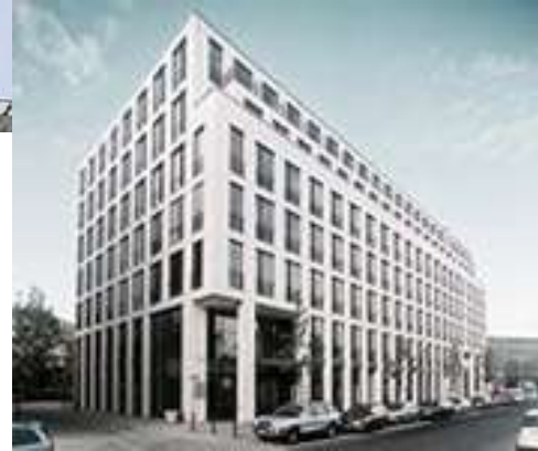
Headquarter Wegelystrasse 3 Berlin
